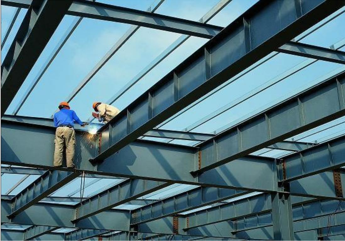
**Project introduction:** The project was a steel-structured two-story workshop with an architectural area of 12,160 m<sup>2</sup> and a designed load capacity of 1,000kg/m<sup>2</sup>. The second floor with an area of 6,000 m<sup>2</sup> was required to be seamless. This hard nut was cracked with joint efforts of both Zhejiang University and our company.
