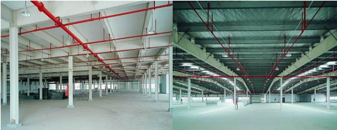
**Project introduction:** This project was a two-story pure steel-structured factory building with an architectural area of 25,000 m<sup>2</sup> and a load capacity of 1,000kg/m<sup>2</sup> on some floors. The factory building, which was a “key-handover” project, looks simple and elegant from the outside and is mainly for manufacturing high quality wooden shutters for exportation.
